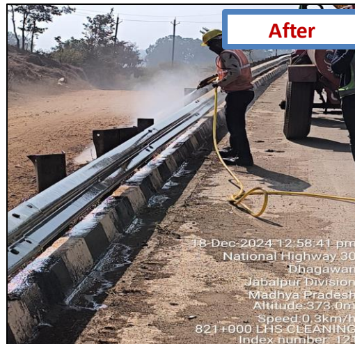
RJKL – Road furnitures cleaning using jet sprayer
